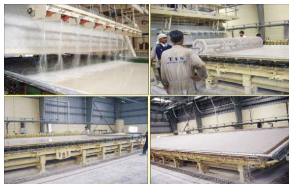
Fig 4 Wall panel plant
