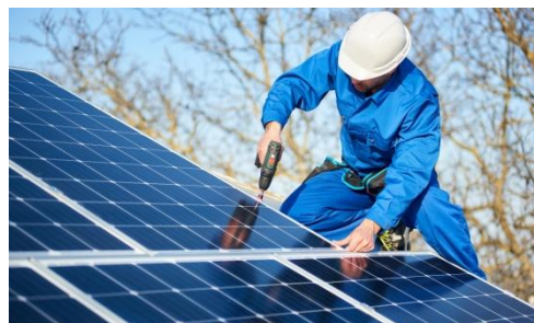
Fig 3 installation of solar panels
