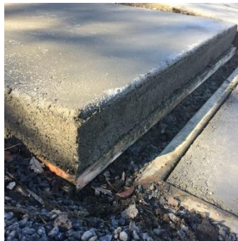
Fig 1 Floating concrete structure
