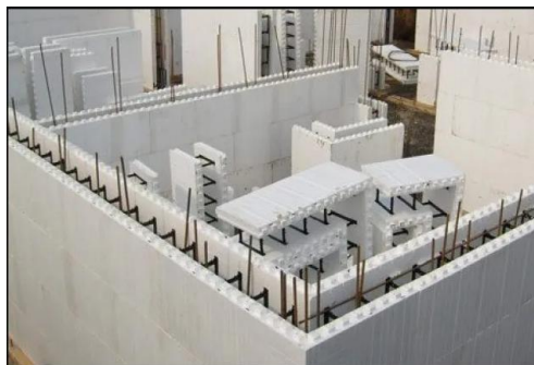
Fig 10 Insulating concrete framework
