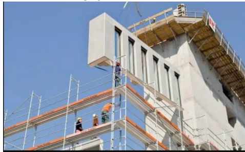
Fig-9 Hybrid concrete construction
