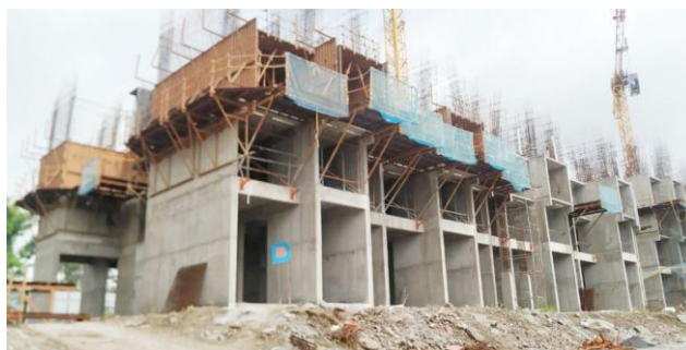
Fig 5 Tunnel formwork system
