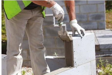
Fig-8 Thin joint masonry technique
