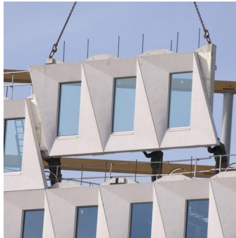
Fig 6 Precast flat panel modules
