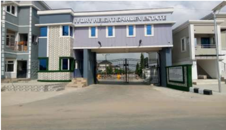
Plate 5: Access Gate of Ivory Height Garden Estate
