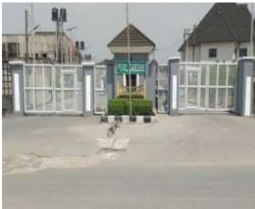
Plate 3: Access to Pearl Gardens Estate
