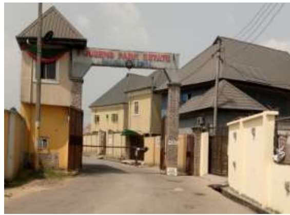
Plate 4: Access to Paradise Park Estate
