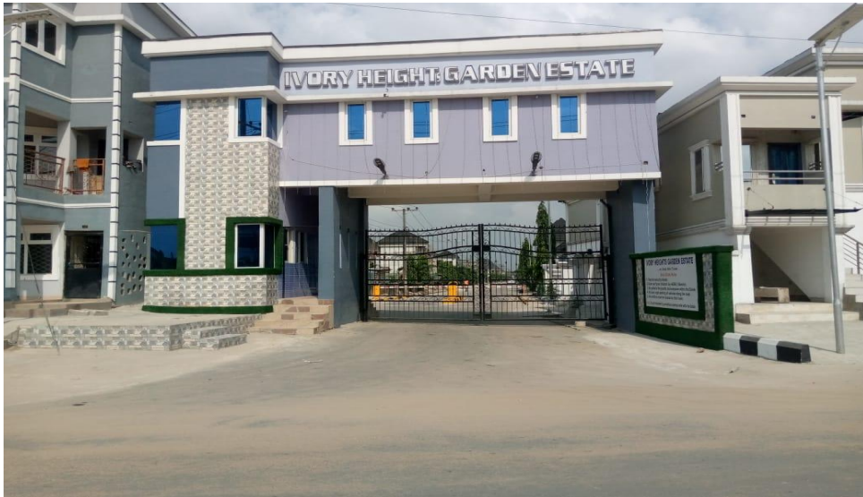
Plate 5: Access Gate of Ivory Height Garden Estate
