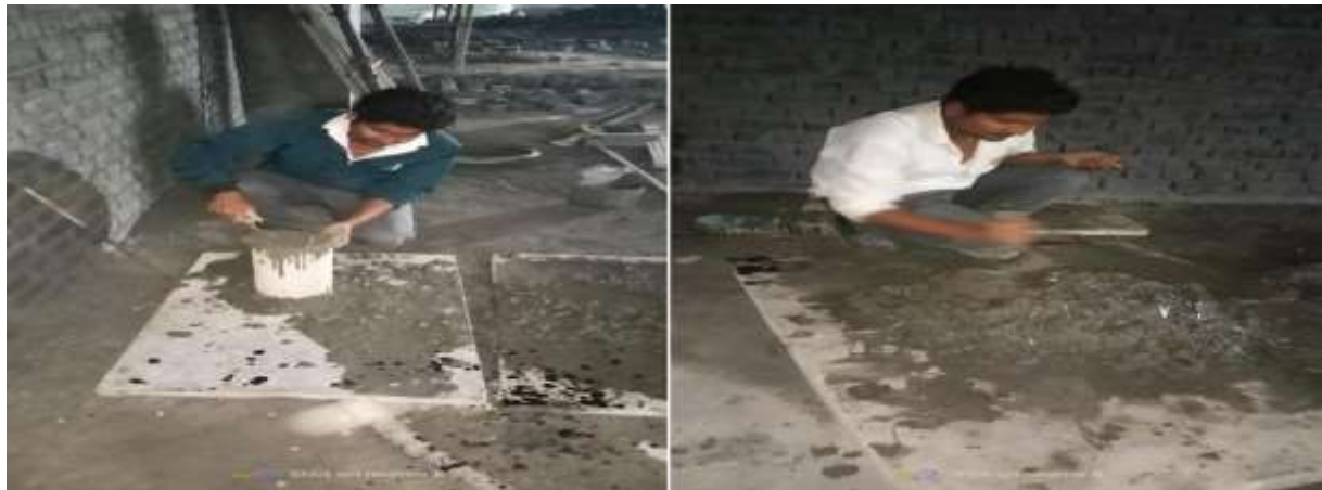
Figure 2 Preparation of concrete cubes
