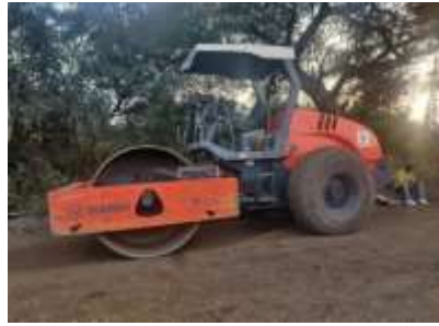
Fig.5 Final layer is properly compacted by soil compacter
