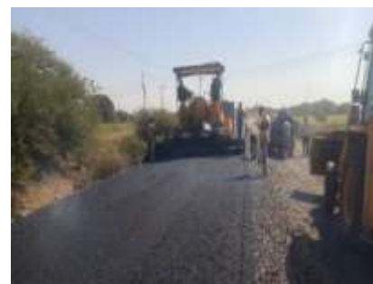
Fig.6 Bituminous Concrete laying Laying
