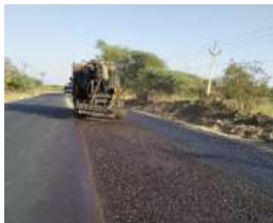
Fig.5 Tack coat spreading
