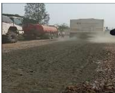
Fig.1 Cement Spreading
