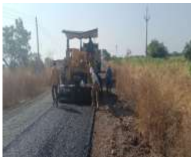
Fig.4 Dense bituminous macadam
