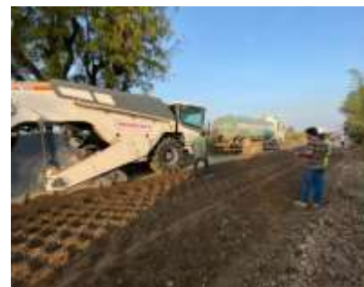
Fig.2 Mixing with CTSB machine
