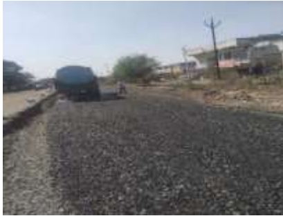
Fig.1 Granular Sub-base spread
