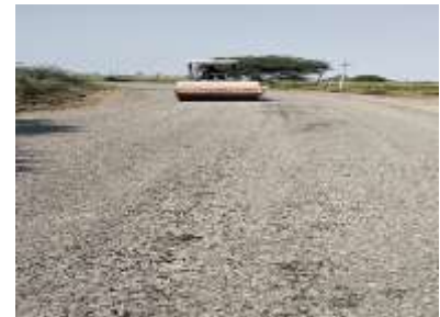
Fig.3 Wet mix macadam spread and compact
