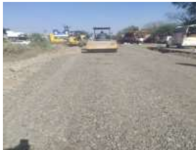
Fig.2 GSB compaction
