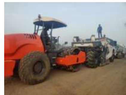
Fig.3 Compacted using sheep foot vibratory roller
