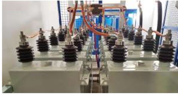
Fig 1: Connections of Capacitor Banks
