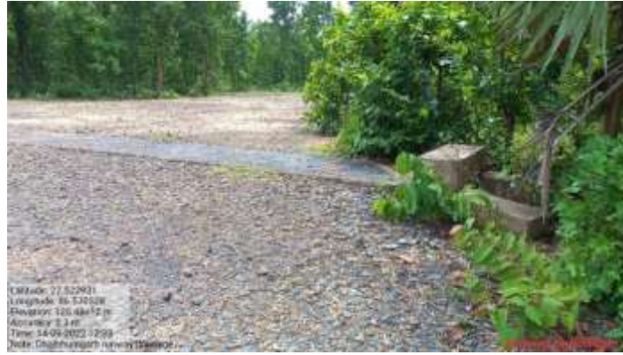
Figure 1.7: Culvert constructed across pavement, Dhalbhumgarh
