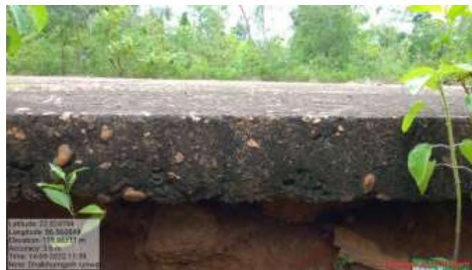
Figure 1.5: Cross-section view of runway, Dhabhumgarh
