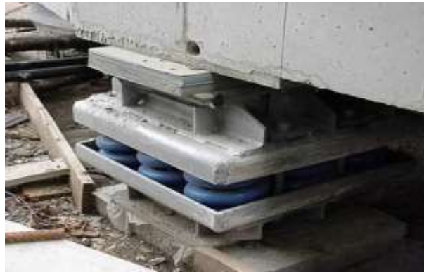
Figure1: Spring Isolators
