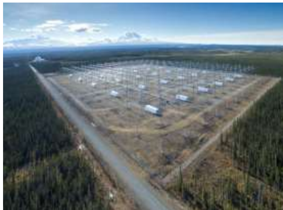
Figure 1. The 180-antenna HAARP array is spread across a 40-acre site at Gakona, Alaska.
