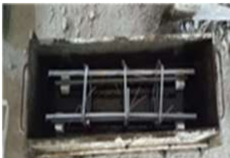
Fig 2-Specimen preparation for CFRP Beams
