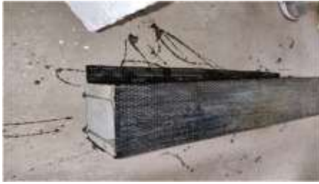
Fig 4-CFRP Strengthened RC Beam (SB-1)
