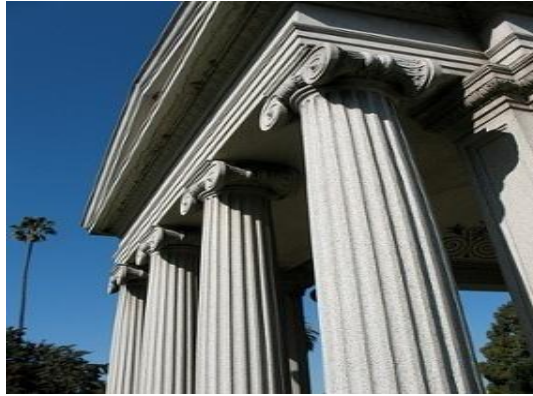
Figure.1.3 Fluted Concrete Columns
