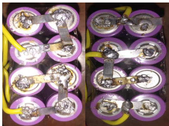
Fig.3.2. Battery Connections (Series and Parallel)
