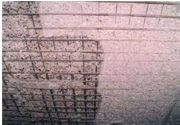
Fire damaged slab
