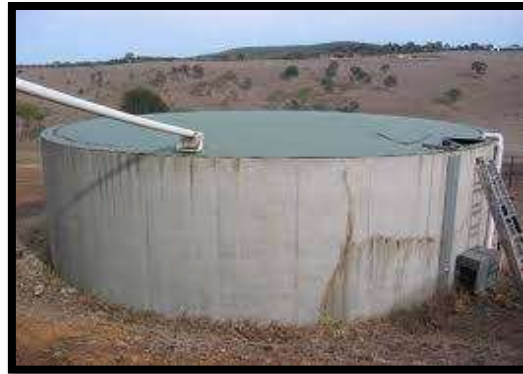
Fig no.1 Water Tank Resting over ground
