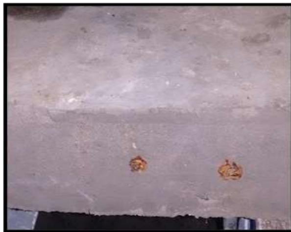
Figure 12- Pattern of crack in solid slab (at 75.2 KN)
