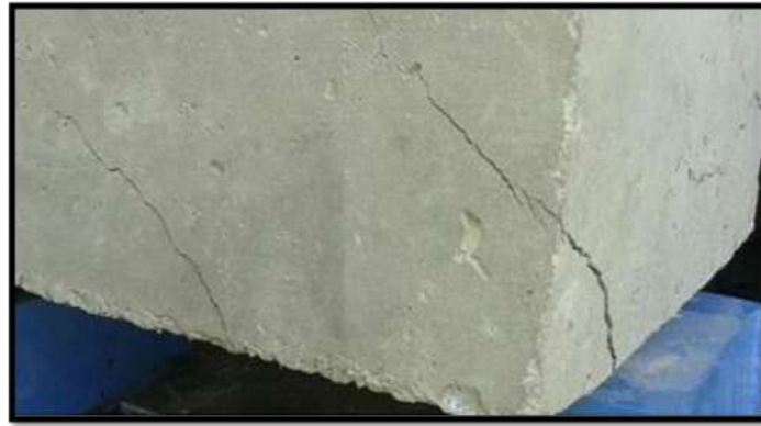
Figure-13-pattern of cracks in bubbledeck slab (at 59.6kN)
