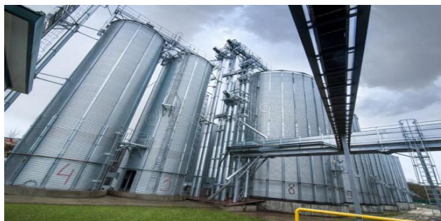
Fig. 1 - Installed tower silos
