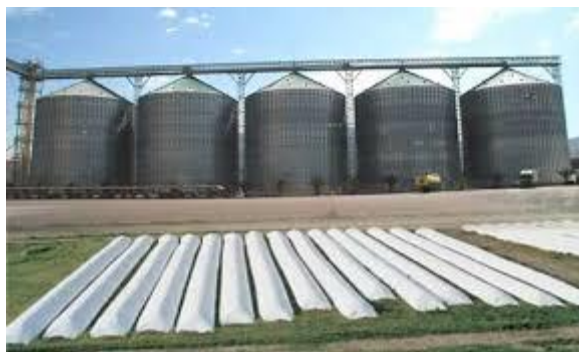
Fig. 3 - Bag Silos for Grain Storage
