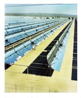
These troughs are lined up in rows on a solar field. A heat transfer fluid is heated as it is run through the pipes in the parabolic trough. This fluid then returns to heat exchangers at a central location where the heat is transferred to water, generating high-pressure superheated steam. This steam then moves a turbine to power a generator and produce electricity. The heat transfer fluid is then cooled and run back through the solar field.
