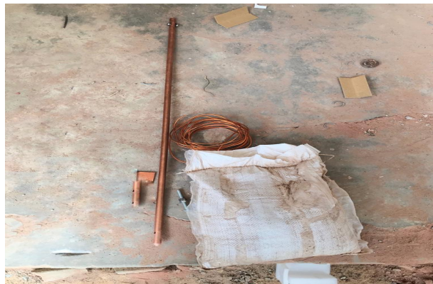
Fig-3: Rod Earthing
