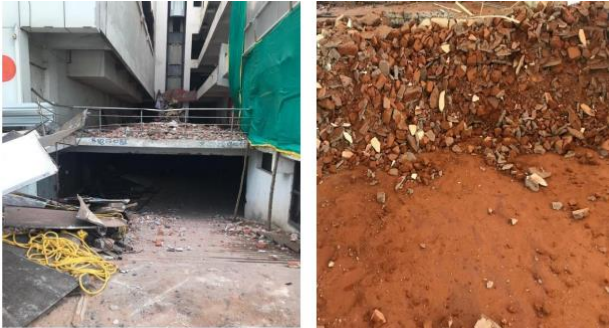
Fig. no.1 Demolition site near Hanamkonda bus stand, Warangal
