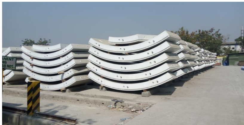
Fig.5: Wadala Segment Casting Yard
