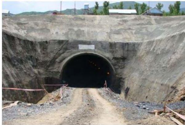
Fig.1. NATM Portal Face Entrance
