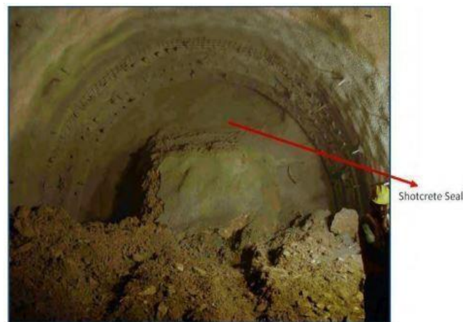
Fig.10.NATM in Action, Shotcrete the end of section
