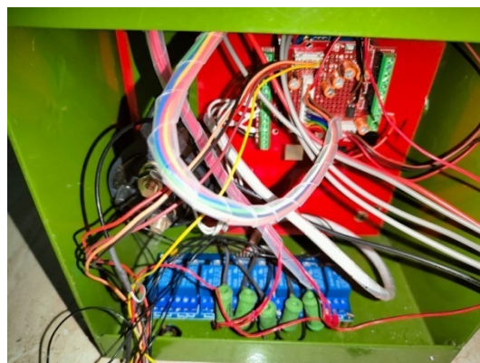
FIG. 9 -Entire BMS setup
