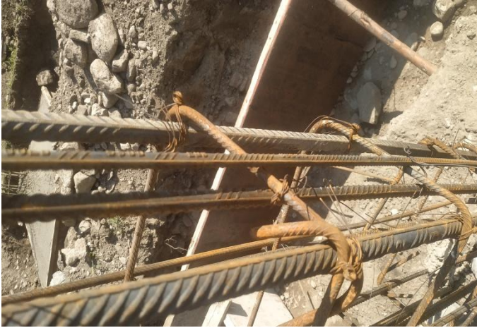
Fig 8 (Improper Reinforcement)
