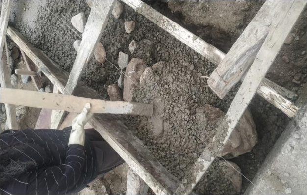
Fig 2 (Segregation of Concrete) Fig 3 (Excessive Plums in Concrete)
