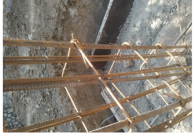
Fig 9 (Reinforcement Bar outside Ring)
