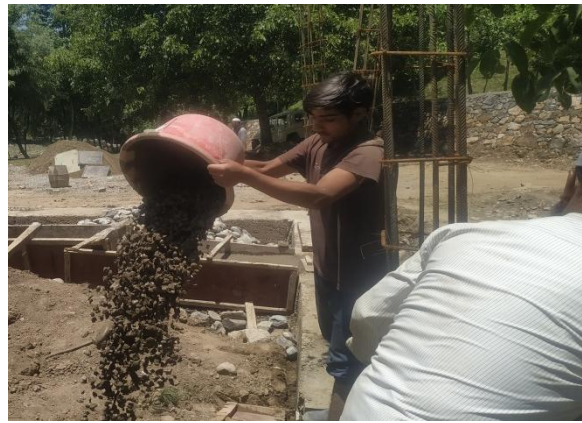
Fig 5 (Dropping Concrete from High Levels)
