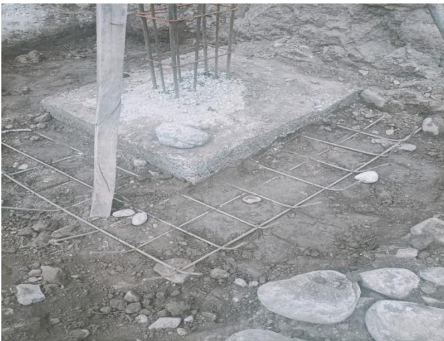
Fig 10 (No Bend provided in Reinforcement)
