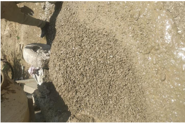
Fig 4 (Segregation of Concrete)
