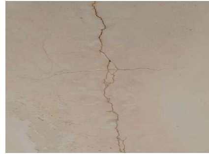
Fig no. 2 Crack on Slab Type- Structural Crack Shape - Vertical Width- 1mm Length- 1000mm Cause- Due to improper curing and thermal variation
