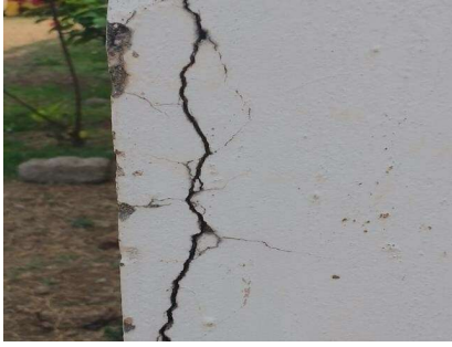
Fig no. 1 Crack on Column Type- Structural Crack Shape - Vertical Width- 2mm Length- 420mm Cause- Due to clear cover
