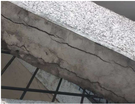
Fig no. 1 Crack on Column Type- Structural Crack Shape - Vertical Width- 2mm Length- 420mm Cause- At the bottom developed
