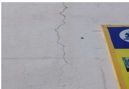
Fig no. 1 Crack on Column Type- Structural Crack Shape - Vertical Width- 2mm Length- 420mm Cause- Thermal variation
