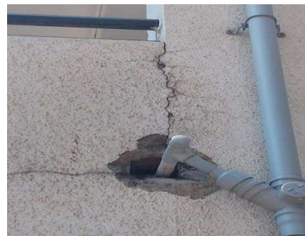
Fig no. 2 Crack on Slab Type- Structural Crack Shape - Vertical Width- 1mm Length- 1000mm Cause- Due to plumbing operation tensile and flexural stresses
