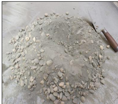
Fig; Mixing of concrete
