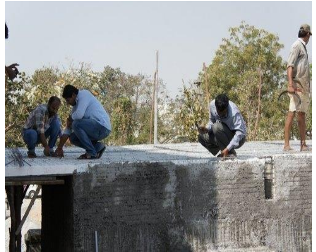
Fig no. 3.2 Construction of Floor in EPS panel
