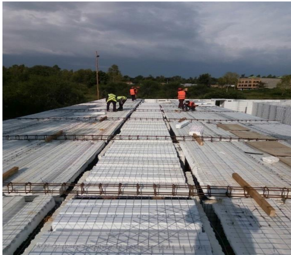
Fig no. 3.2 Construction of Floor in EPS panel
