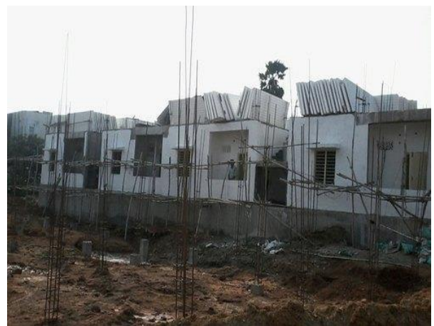
Fig no. 3.1 construction of EPS wall panels in load bearing structure
