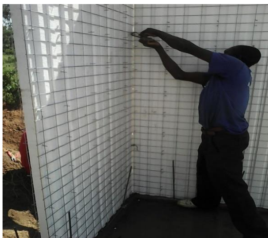
Fig no. 3.1 construction of EPS wall panels in load bearing structure
