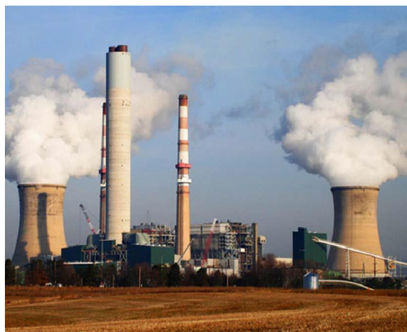
Fig. 1: Self-supporting Steel Chimney
