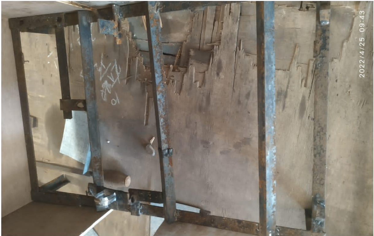
16. The next we have completed that connection to fix the back part of trailer.
