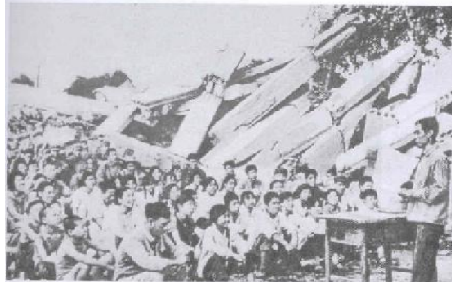
Fig 14 Collapse of precast buildings
