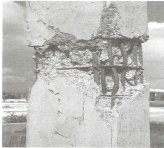
Fig -16: Close-up of poor column details
