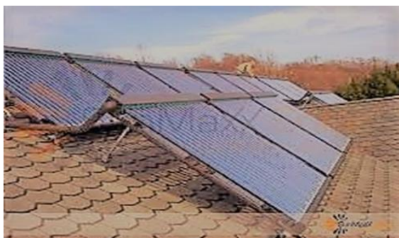
Fig.3 Evacuated tube collectors
