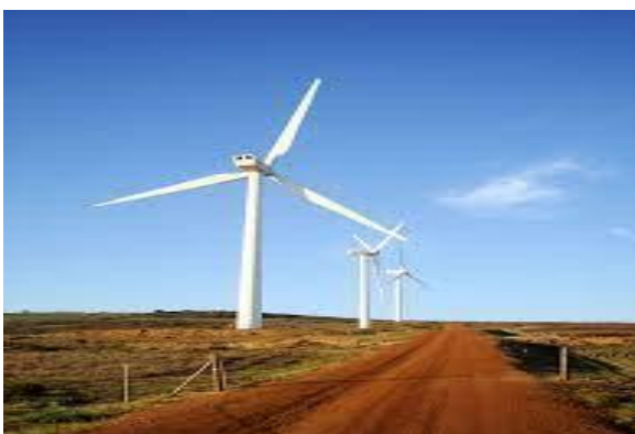
Fig. Wind turbine
