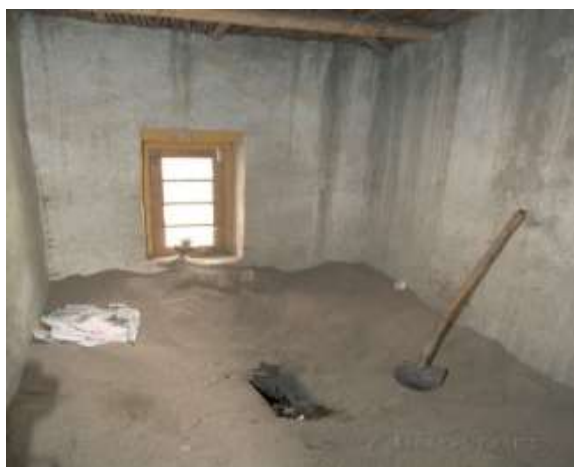
A typical traditional toilet in Ladakh
