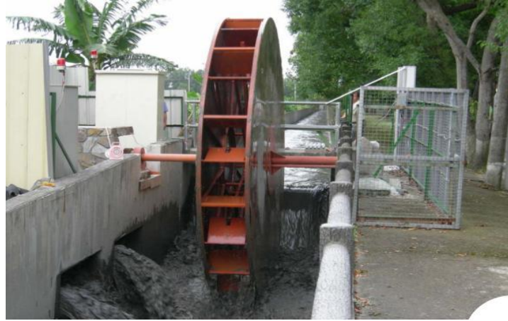
Fig 8 :Micro Hydro Power Generation System
