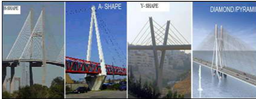
Fig.3: Different Shapes of Pylons
