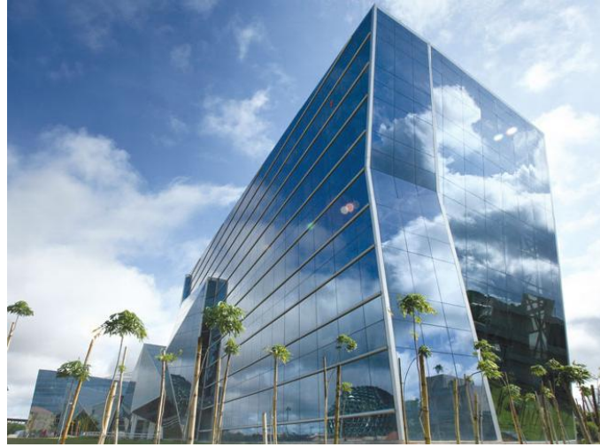
Fig. 2 – The Structure Reflects The Site's Rugged Contours.
