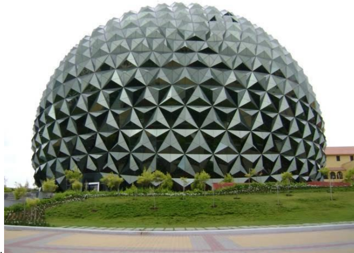
Fig. 4– The Dome Shaped Multiplex & Auditorium
