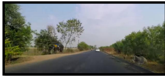
Figure 5.1: Problem Identification at chainage CH 2.8 (Ghatol)
