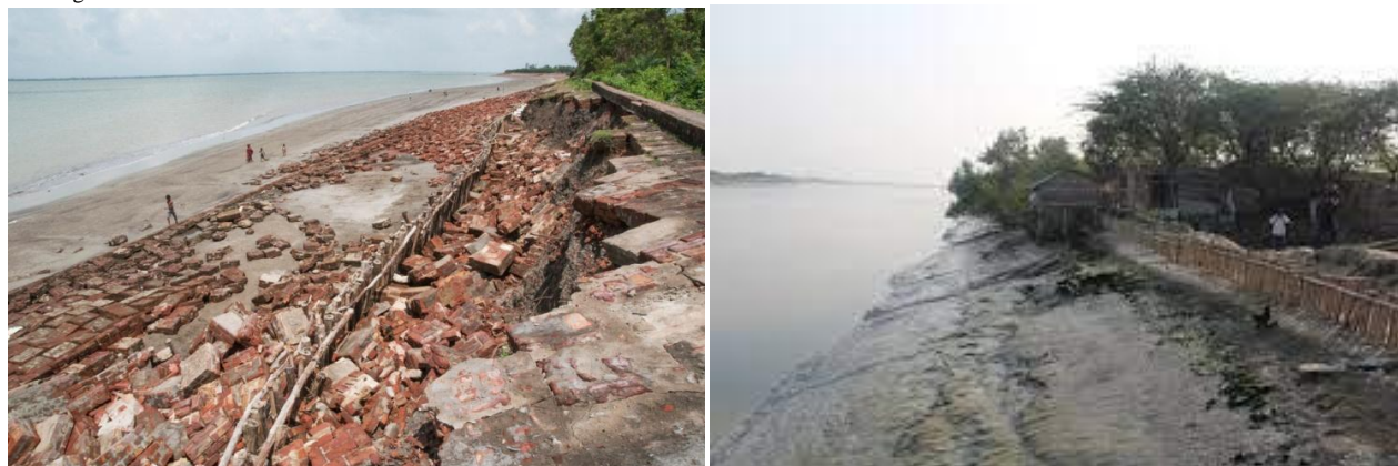
Dams of Sundarbans after Aila. Renovation going on.
