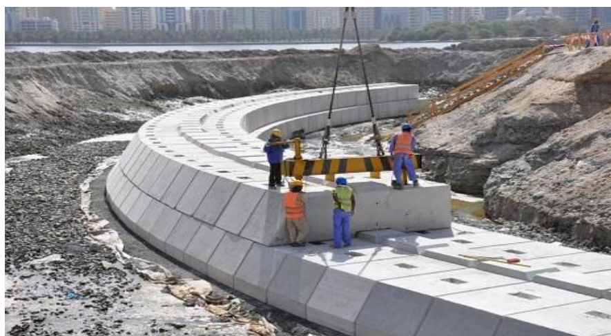
Fig 12: Gravity block quay walls.
