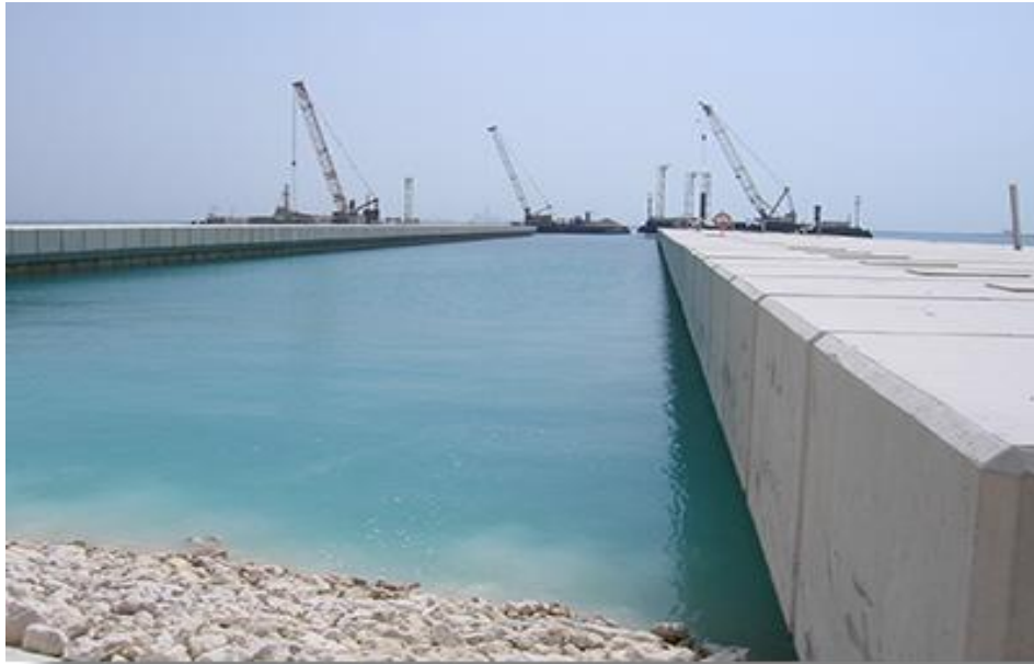
Fig 13: counterfort quay walls.
