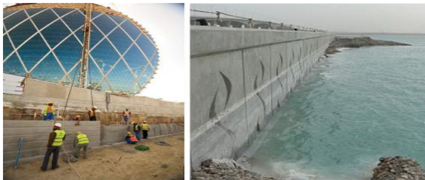
Fig 11: Diaphragm walled quay walls.
