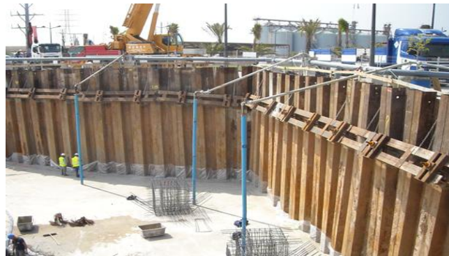
Fig 8: Sheet piled quay walls.
