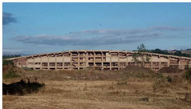
Fig.3 Construction Site in the study area
