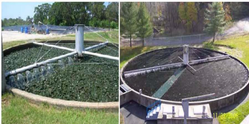
Figure - 9: Trickling filter
