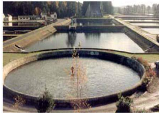
Figure -19: Sewage oxidation ponds
