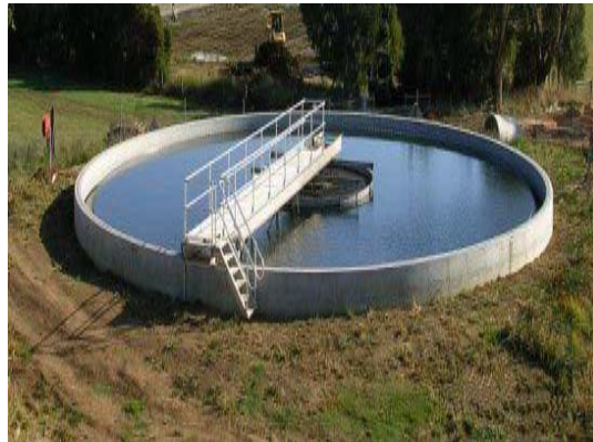
Figure 6: Primary settling tank
