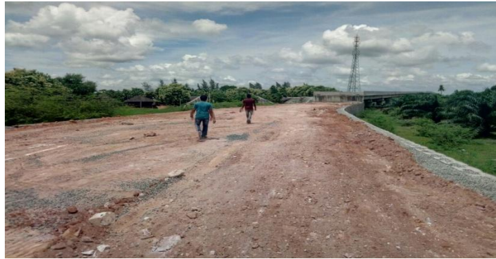
Fig 1.2: Present condition of yarraguntla -proddutur road
