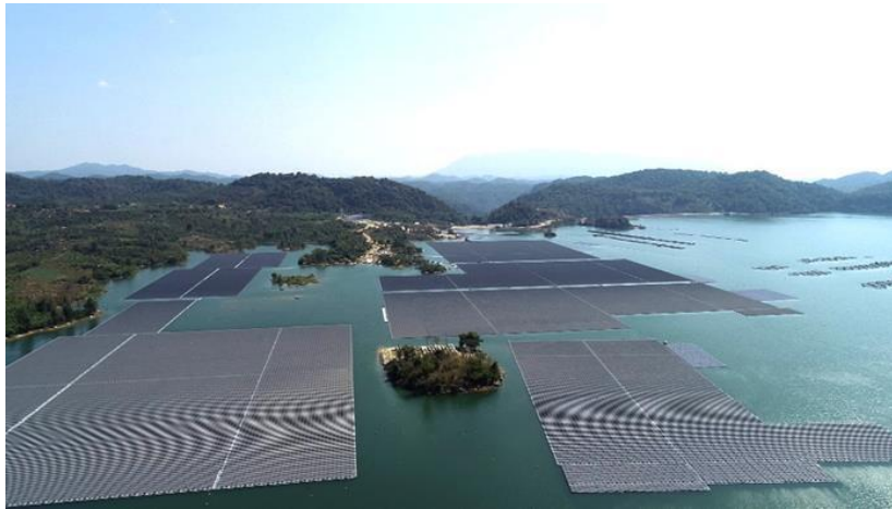
Figure 3-Solar Panels Installed on Da Mi Hydroelectric Reservoir (Source - (Evn, 2019))
