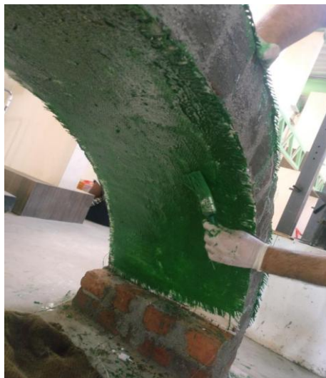
Fig 6: Application of GFRP on intrados
