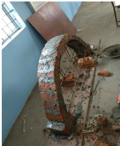
Fig 3: Casting of brick arch
