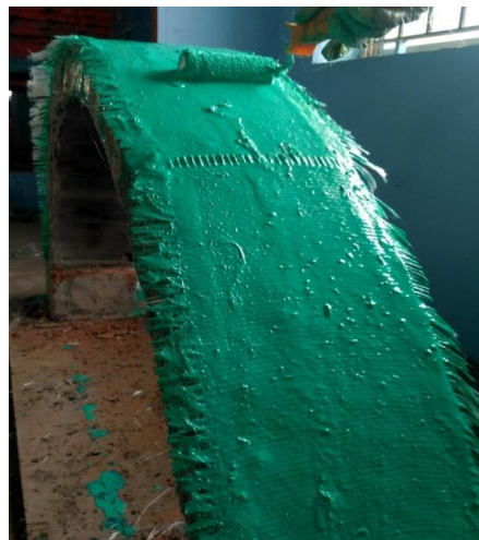
Fig 5: Application of GFRP on extrados
