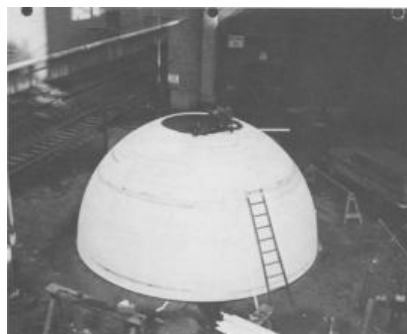
Fig. 27 - A 30 ft. (9.15 m) Diameter Styrofoam Dome, 2 in (50 mm) Thick, Nearing Completion
