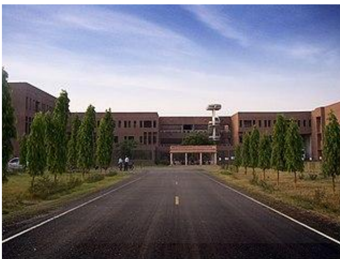
Fig1. This Photois of Flexible pavement IET Lucknow.
