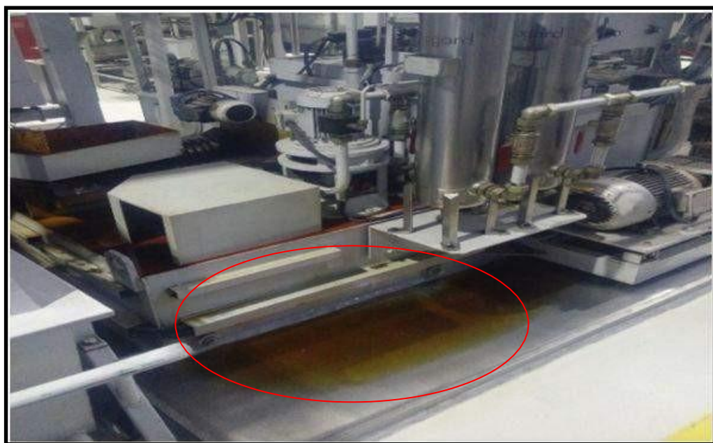
Fig. 1.2.2 Overflow Due To Chips Clogging
