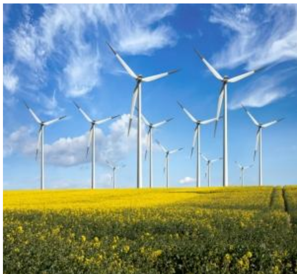
Fig 4. Windmills constructed in between the fields
